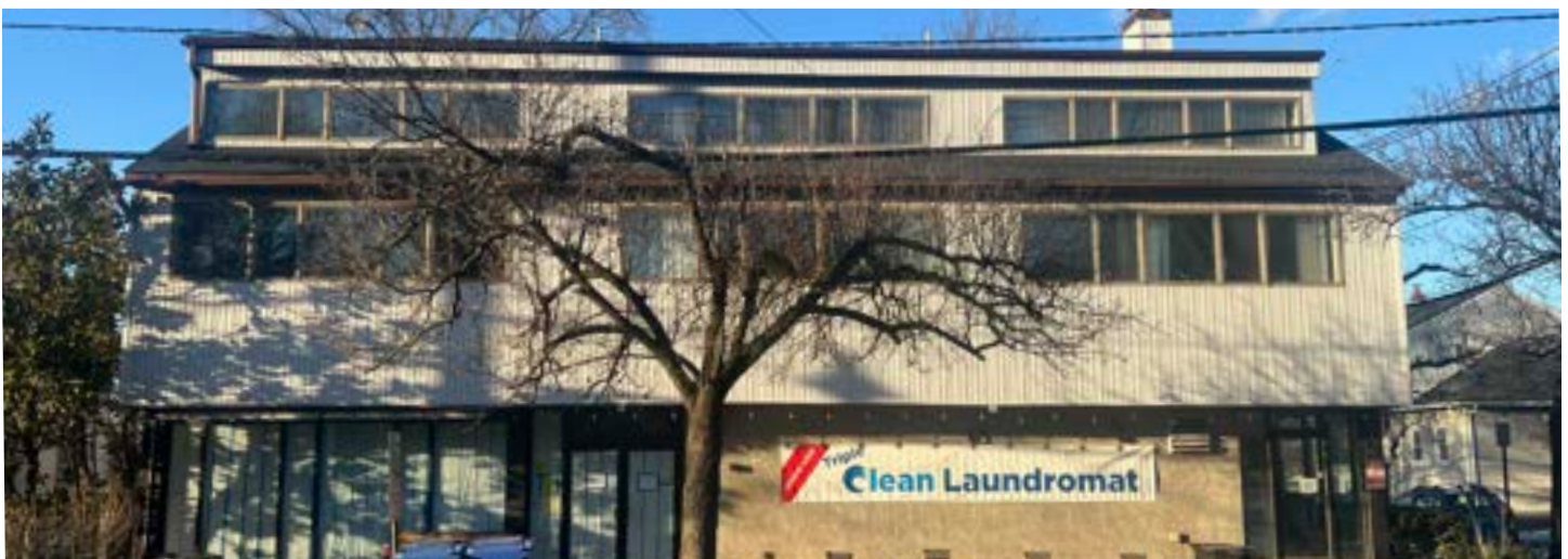
Highland Park Laundry: After
