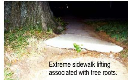
Extreme sidewalk lifting associated with tree roots.
