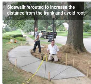
Sidewalk rerouted to increase the distance from the trunk and avoid root
