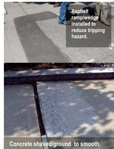
Asphalt ramp/wedge installed to reduce tripping hazard.
